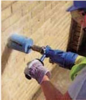
Weka DK1203 is a powerful 110V 1.5kW 3 speed motor fitted with a heavy-duty centrifugal clutch. Speed ranges 580/1400/2900. Nose spindle is 1¼"UNC male, with adaptor to ½" BSP female.
