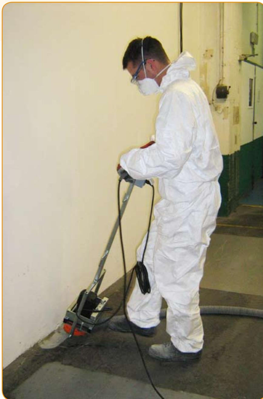
*Cup grinder on use on CG125 grinding machine.*
